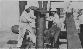
EACH pile was checked for vertical alignment. CADA palo mestier a wordo examiná pa alineacion.
